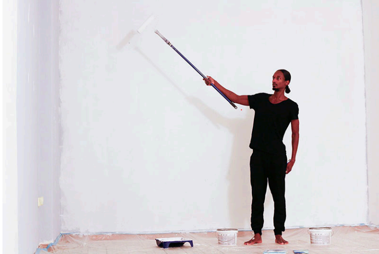
Figure 9.5 A painter uses an extension roller to paint a wall. (credit: "Paint Rollers are effective" by WILLPOWER STUDIOS/ Flickr, CC BY 2.0)
